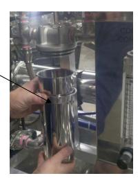
Note: always store your wet RO prefilters in a heated room so they don't freeze. A frozen prefilter will not work.
